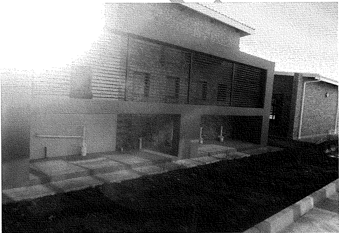
Figure 34 Multipurpose centre community hall
